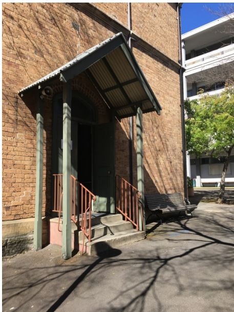
3 Block D: original or early steps, balustrading and timber entry doors and c1990s timber porch are proposed to be removed, in order to accommodate a new accessible entry ramp.
