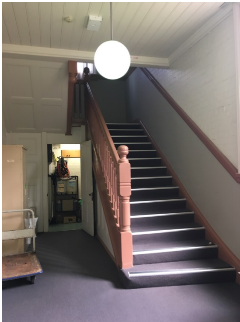
17 Block C: BCA / accessibility upgrade works proposed for the stairs include the addition of compliant handrails and nosings.
